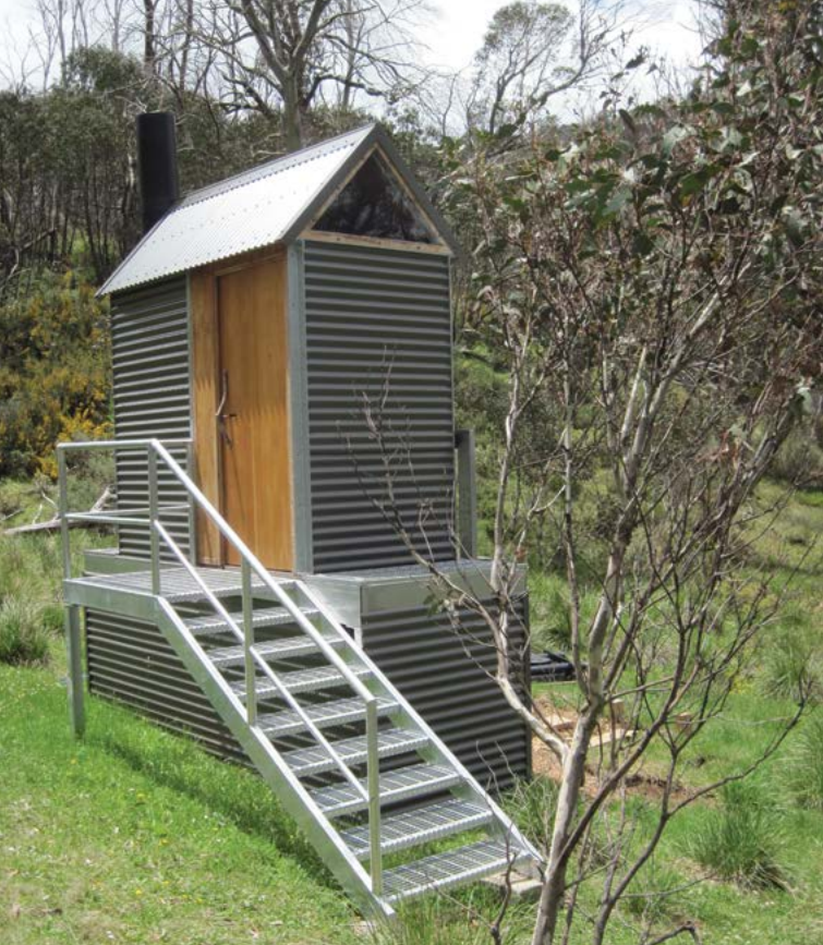
Contemporary-design 'fly-out waste' toilet at Dibbin Hut Camping Area to replace the old earth pit, Alpine National Park, Victoria, Australia
